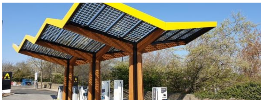
Example solar charging hub in Sunderland.
